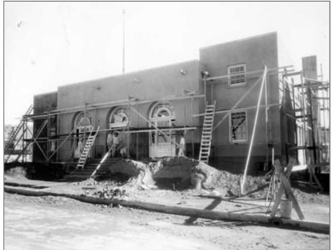
December 30, 1935, Construction photo of front façade of the new U.S. Post Office building at Oak and 4th Street. Stucco and glass and glass door and windows are in place. Sidewalk and curbing are in progress.
