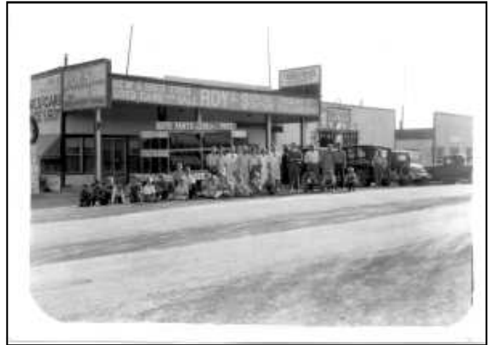
#14514 Roy's Service Station
