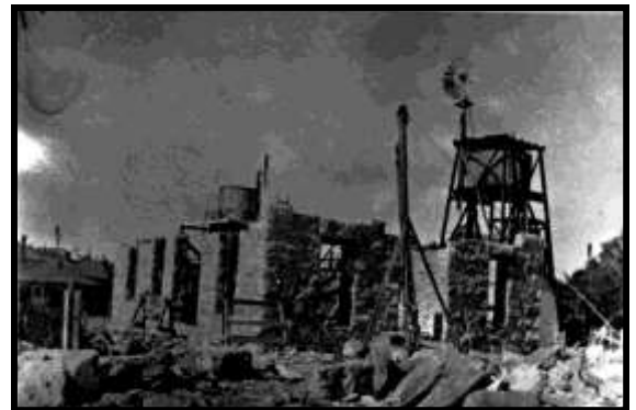
View of Bonelli House under construc- tion in 1915
