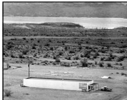
Lake Havasu Plumbing & Hardware, one of 1st commercial buildings completed. Photo taken 2/14/65.
